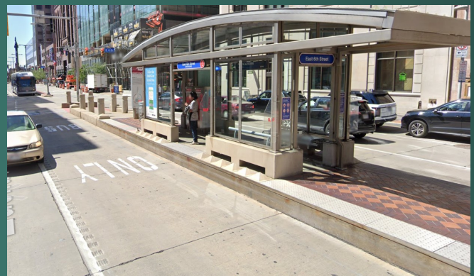
RTA Healthline East Sixth Street Station in Cleveland, OH
